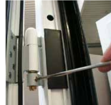
Loosen fixing screw.
